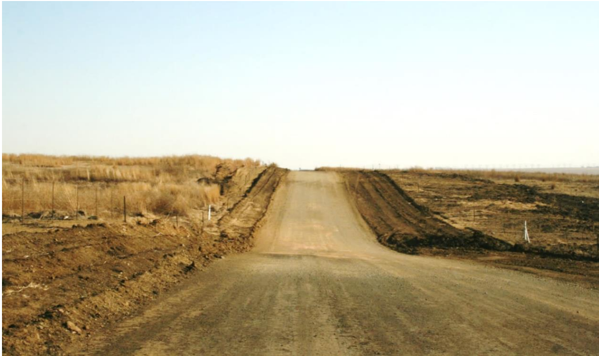
Figure 1(b). Road crossing a longwall mining subsidence trough in flat terrain (source: Hebblewhite, 2022a)
