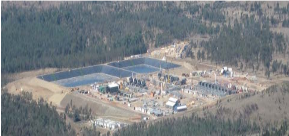
Figure 2: Santos water management facility [6]
